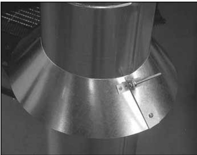
Figure 10.14 Assembling the Storm Collar Around the Pipe
